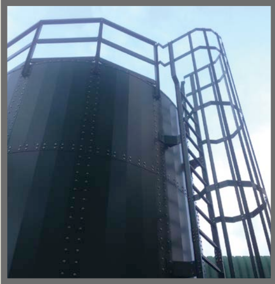
Access Ladder – Including roof access panel
